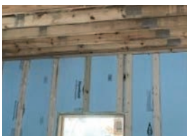
Insulation Insulated wall packages
