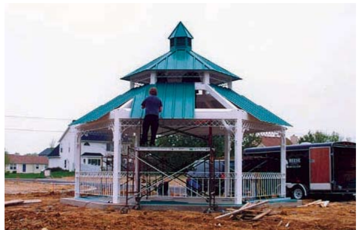
Installation of pre-cut roofing panels
