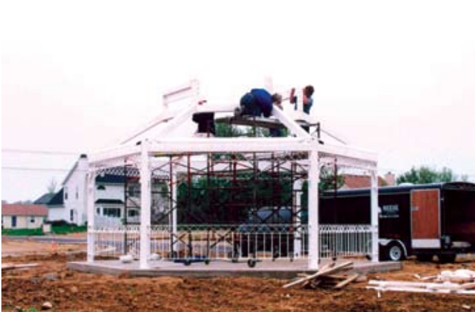
Railing and ornamentation are installed with the frame
