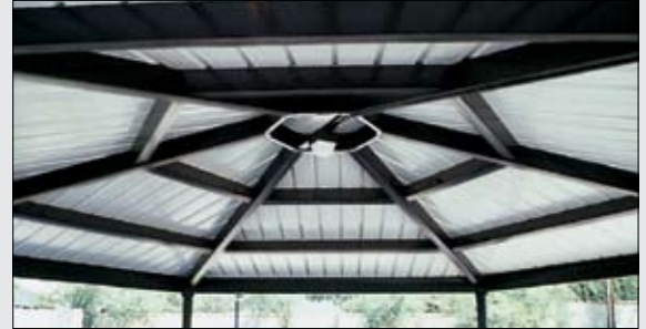
Ribbed Metal Roof Ceiling
