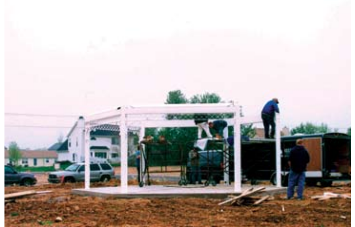
No field welding is required during erection
