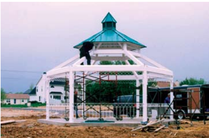
The upper roofing is installed then the cupola
