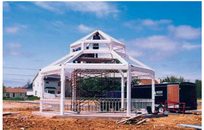
Frame is complete and ready for roofing
