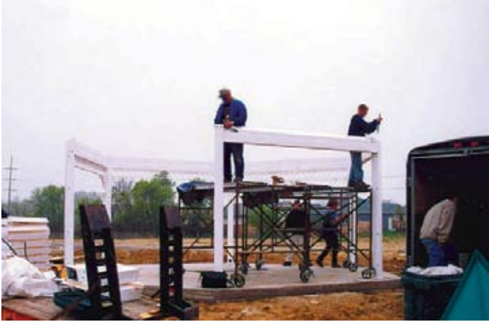
Frames are easily bolted together with provided fasteners
